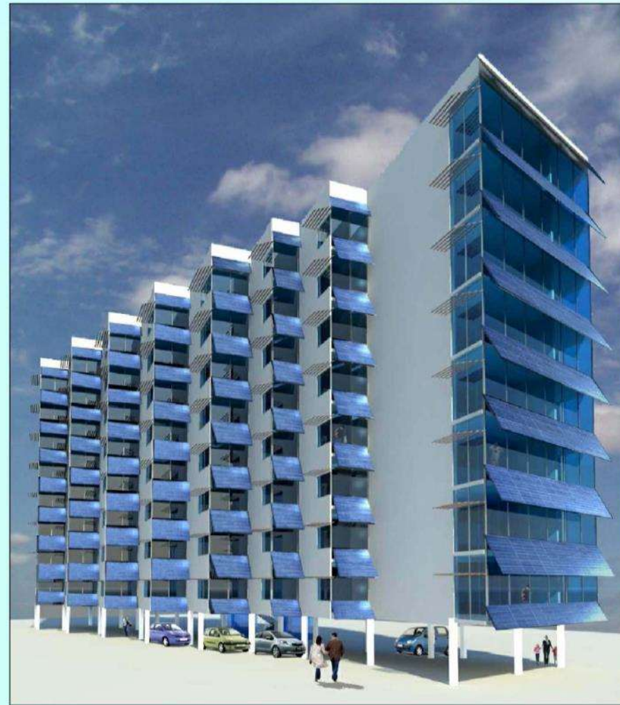
SOUTH - WEST VIEW
